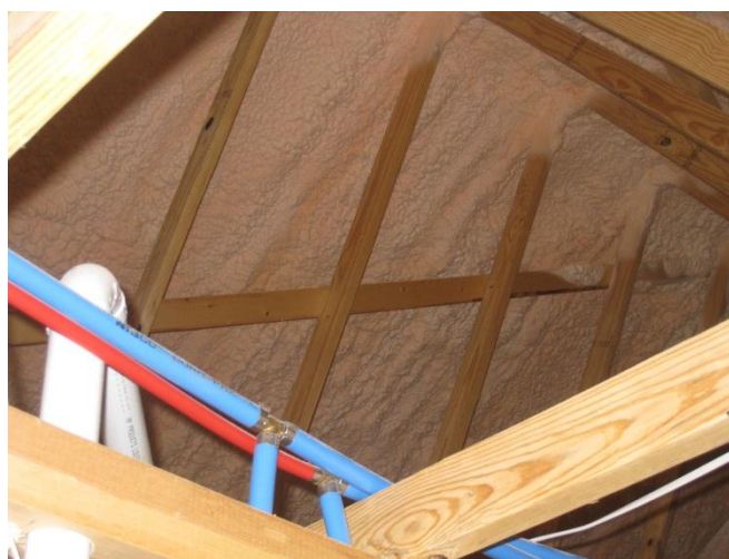
Figure 2 - Spray Foam under a Roof Deck
