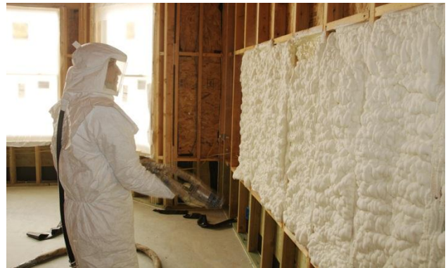
Figure 4 - Spray Foam in an Exterior Wall Cavity
