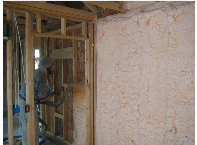
Figure 3 - Spray Foam being applied to an Exterior Wall Cavity
